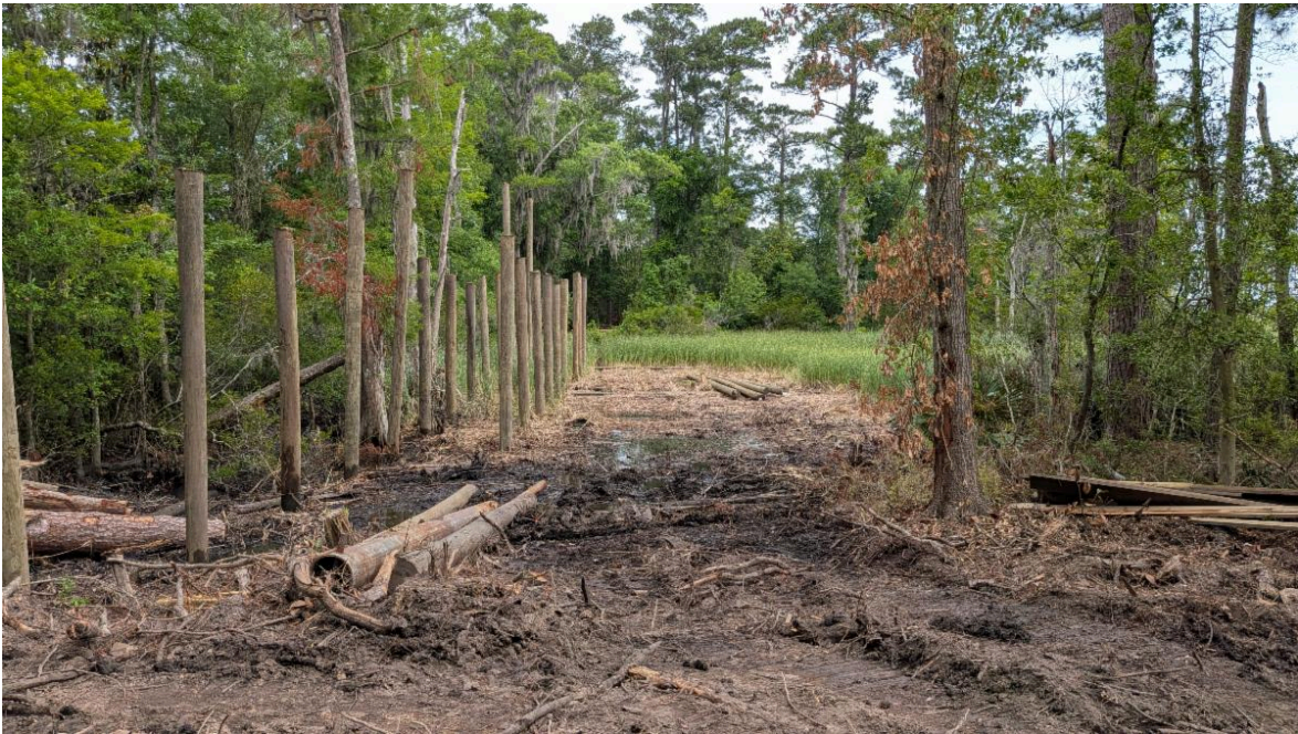
Pylons have been placed along the path where the boardwalk extension will be connected into.
