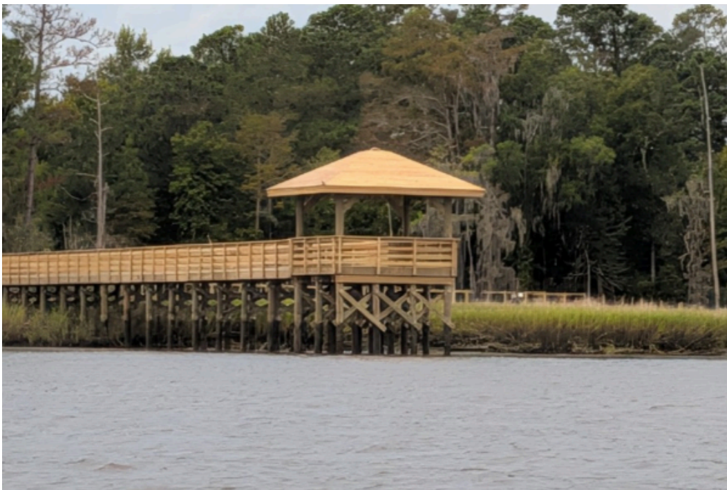
The completed boardwalk extension and gazebo as seen from the Brunswick River. Thanks to our marine contractor, TD Eure for the amazing work.
